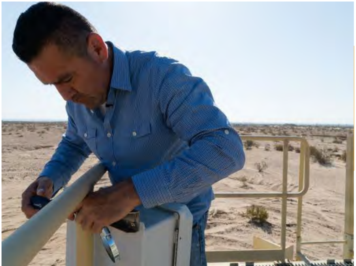
Humberto Lugo of Comite Civico del Valle installs a monitor near the Salton Sea. Each monitor installation is unique and may require different tool or materials. Photo courtesy of Zoe Meyers/The Desert Sun.
